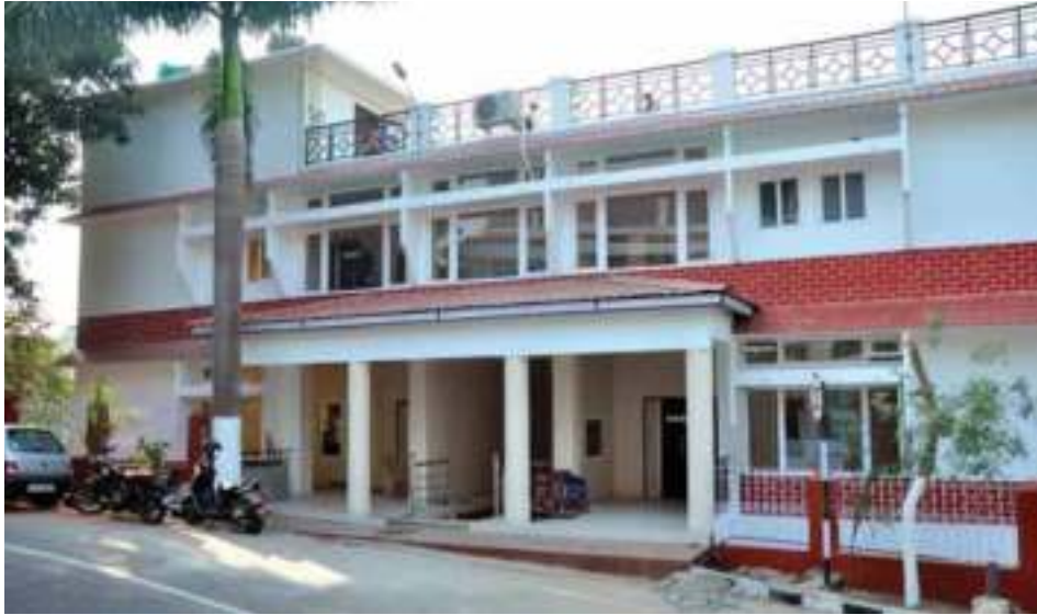
Newly constructed Governor's Secretariat and digital library
