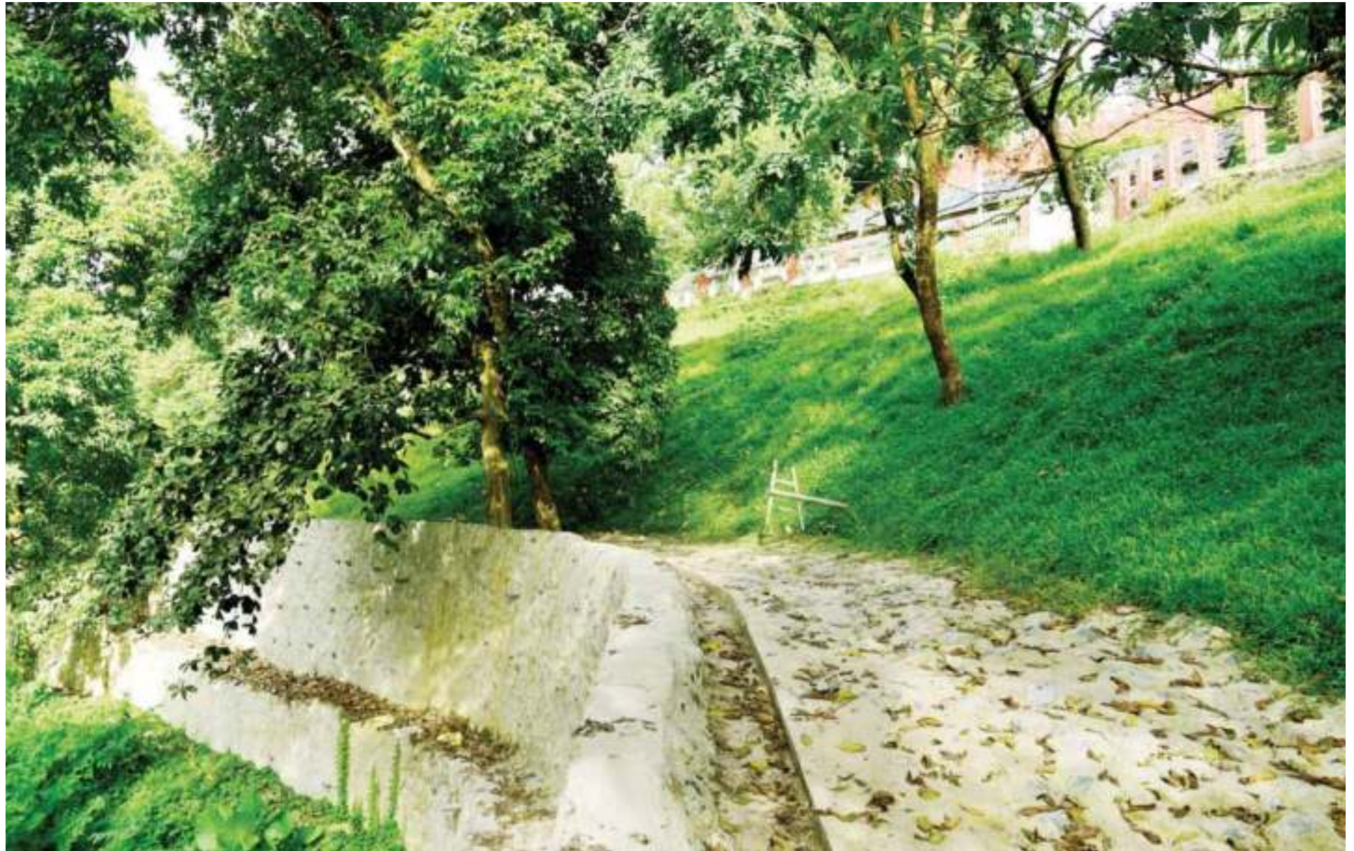
Retaining wall for slope stabilization was constructed at Raj Bhavan
